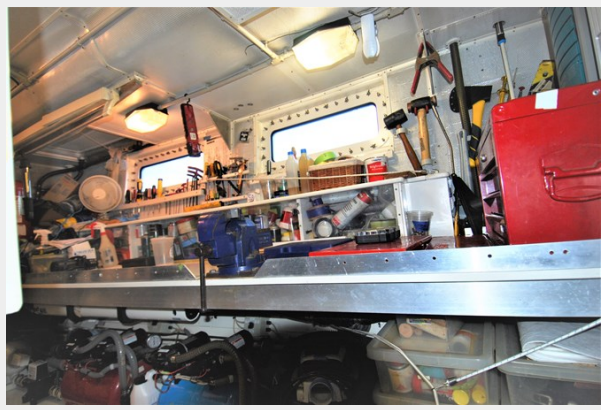
leonore - Port Engine Room
