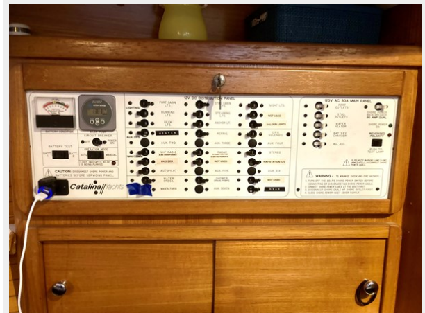
Ships Main Breaker Panel
