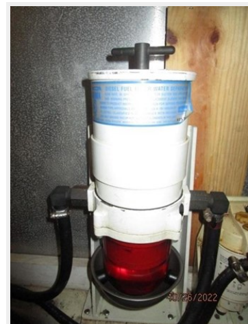
59_2794170_46_carver_port_racor_fuel_filter
