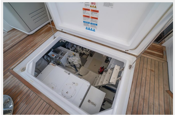
Engine Room Access
