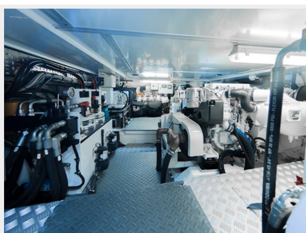
enso engine room
