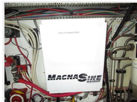
69_2794527_44_defever_inverter_charger
