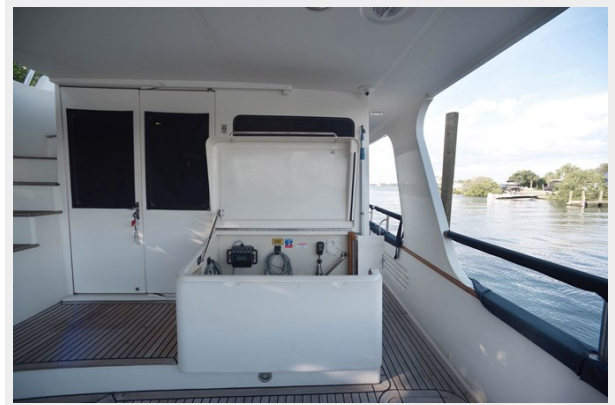
Engine Room Access
