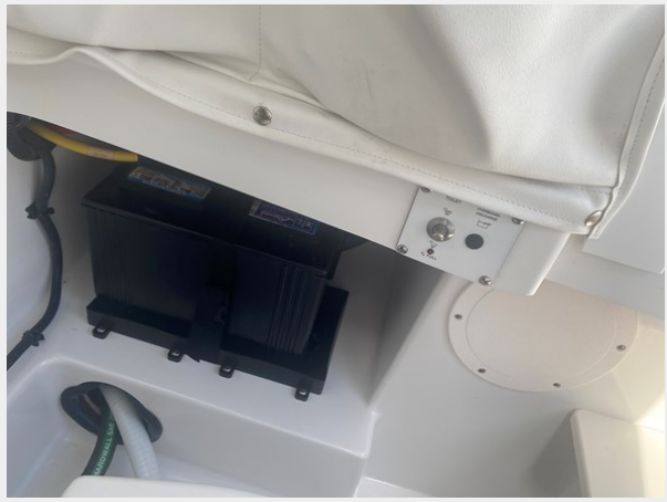
29-Head Overboard Discharge
