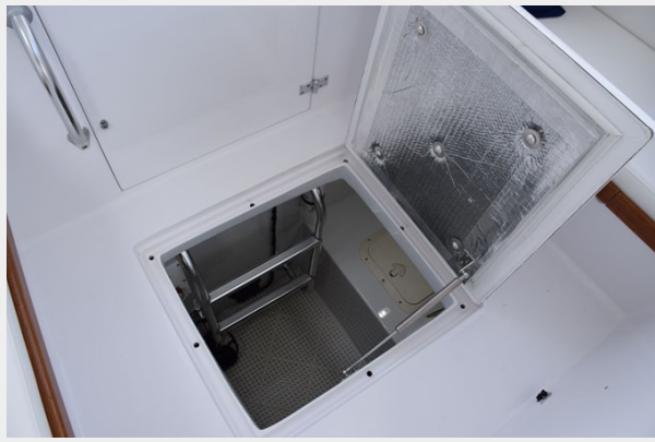
050 Engine Room Entrance Hatch Forward of Helm
