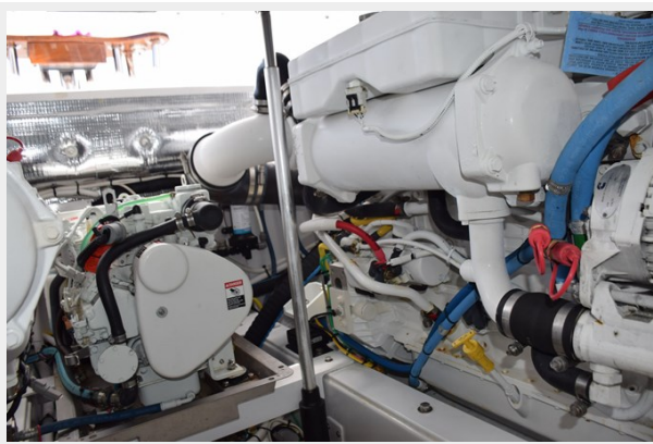
Port Motor and Northern Lights Generator
