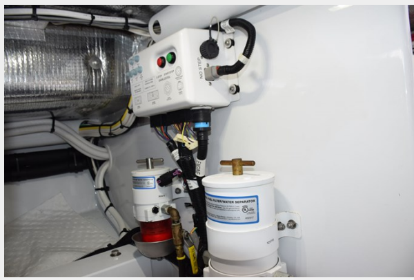
Forward Portside Engine Room, Racor Primary Fuel Filter
