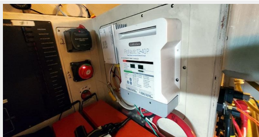
50_2795381_battery_charger_12_vdc
