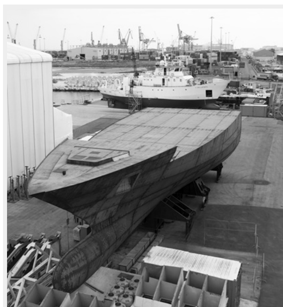
ISA CONTINENTAL 80 under construction
