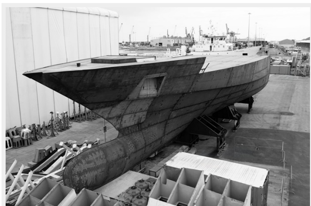
ISA CONTINENTAL 80 under construction
