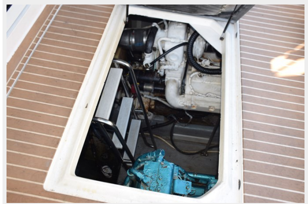
Engine Room Entry Hatch
