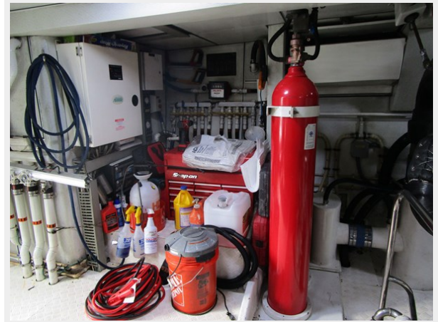
Port Aft Engine Room
