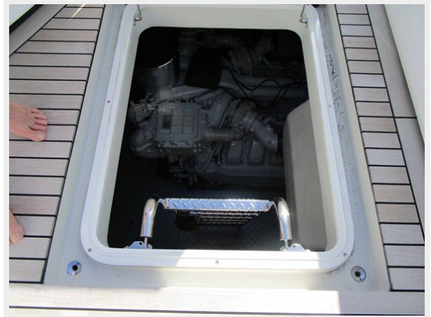
Engine Room Entrance
