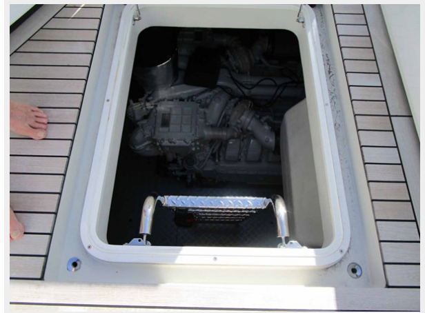
Engine Room Entrance
