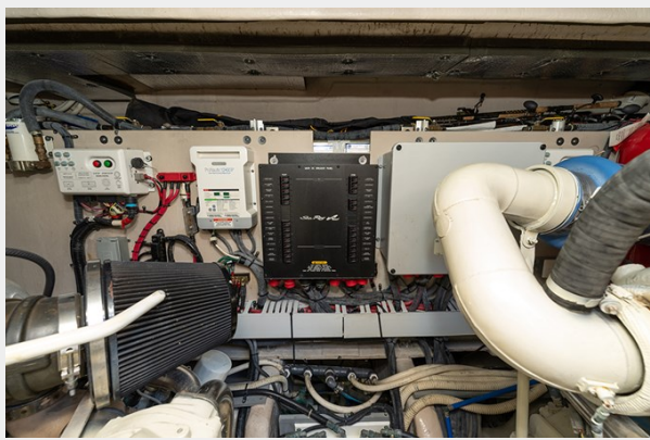
Main DC breaker panel
