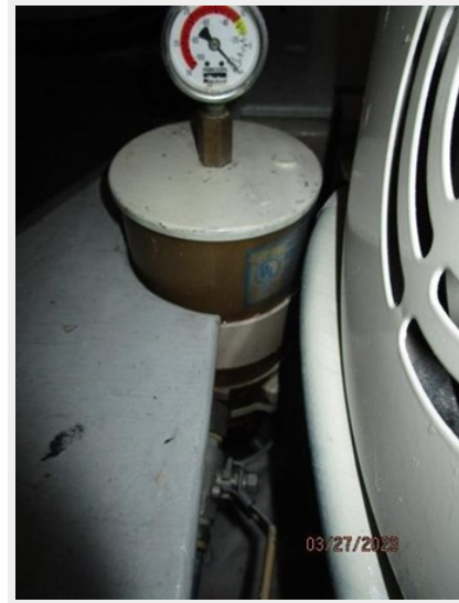
47_2797661_36_racor_fuel_filter
