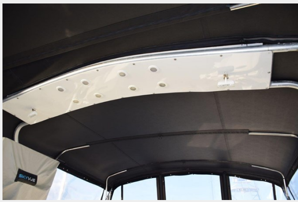
Underside of Flybridge Arch with LED Lighting
