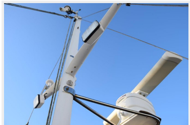
Antenna Mast, Spreader Lights, and Camera
