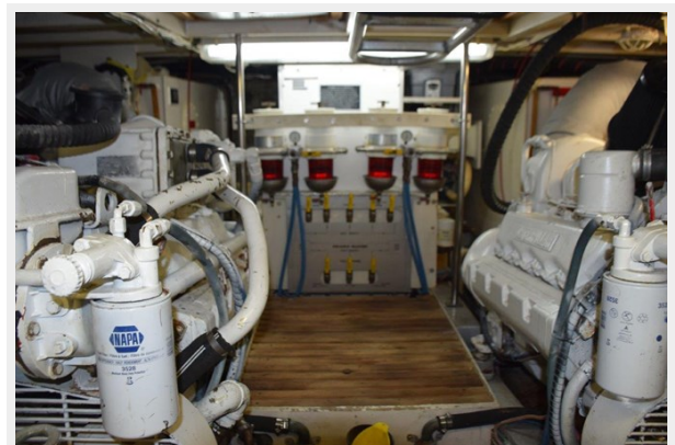
Twin 3208TA CAT Diesels
