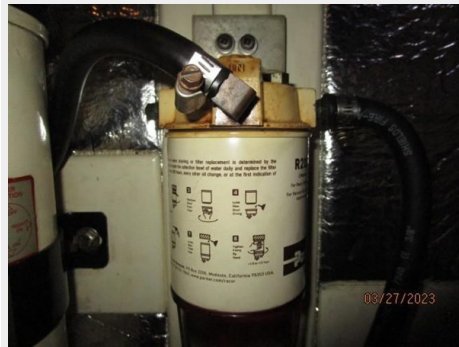
60_2797740_36_heritage_east_generator_racor_fuel_filter
