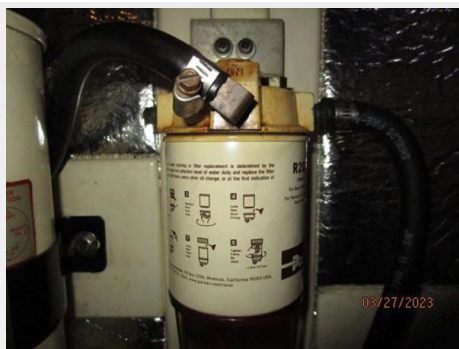
60_2797740_36_heritage_east_generator_racor_fuel_filter
