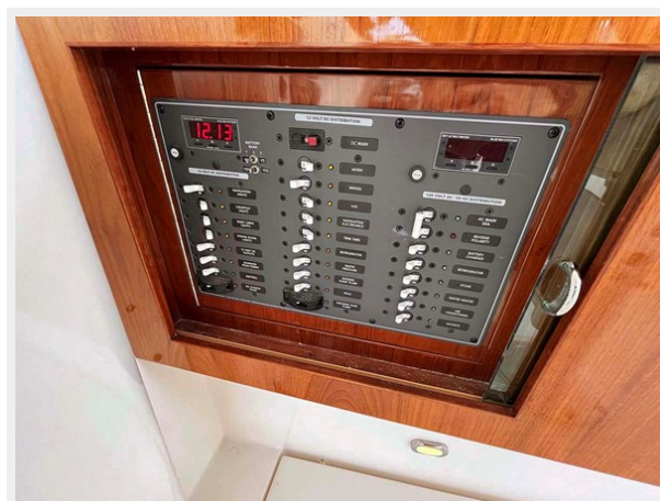
Electrical Panel at Helm
