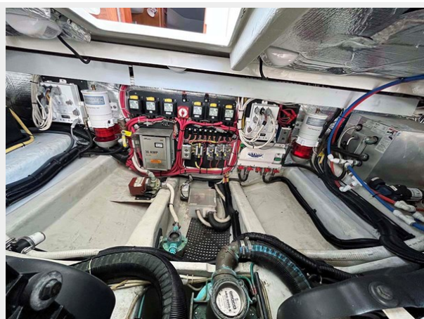
Engine Room Forward
