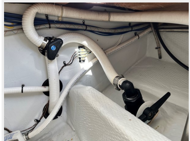
Holding Tank Y Valve
