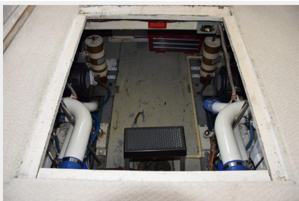
Engine Room Opening
