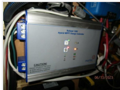
79_2799978_53_bruce_roberts_wind_generator_controller
