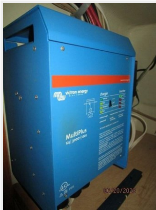
72_2800174_42_kelsall_inverter_charger
