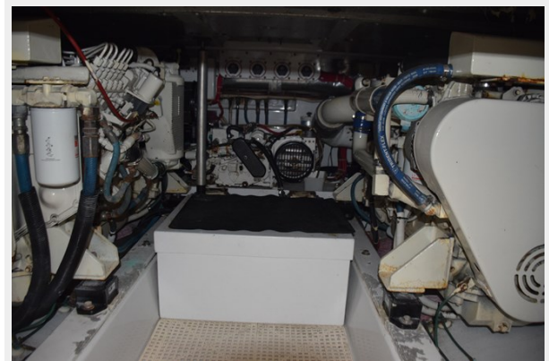
Engine Room, Generator in Center Aft
