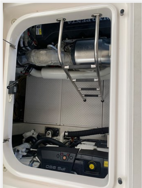
Engine Room Access
