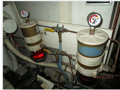
57_2800368_42_grand_banks_port_racor_fuel_filters
