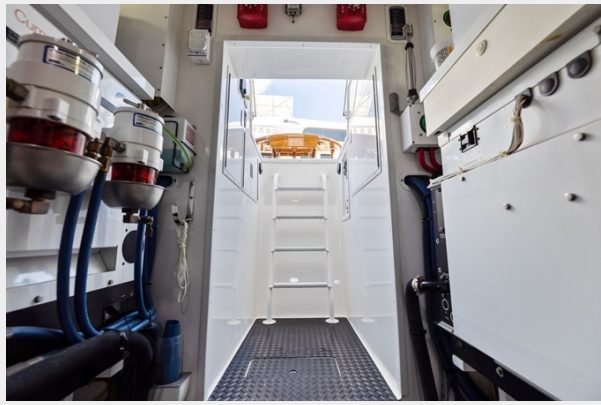
Entry to Engine Room
