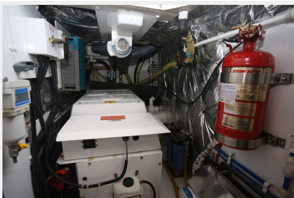
Princess 62 Engine Room
