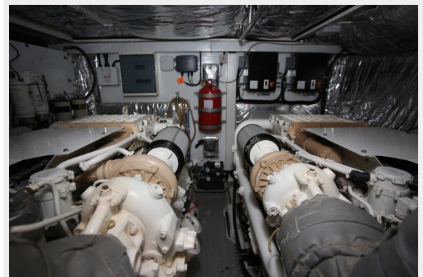
Princess 62 Engine Room
