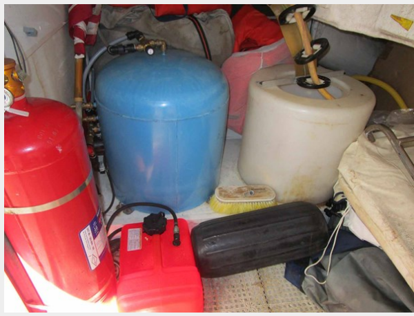
New Water Heater
