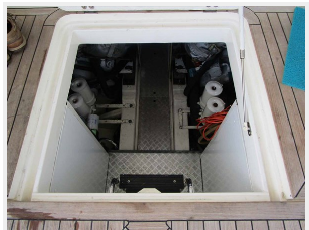
Engine Room Entrance
