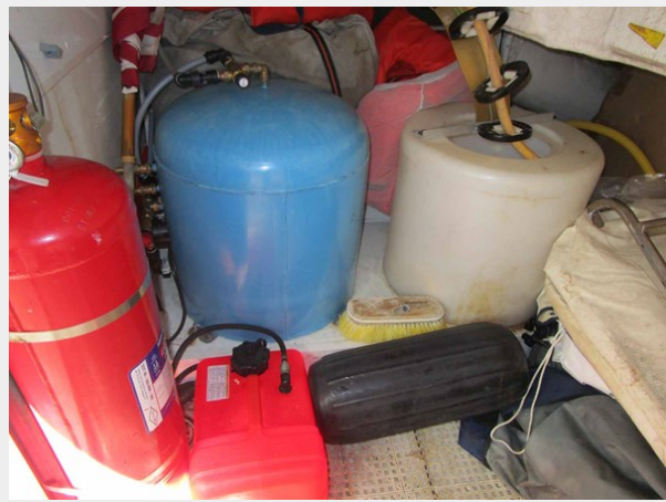
New Water Heater
