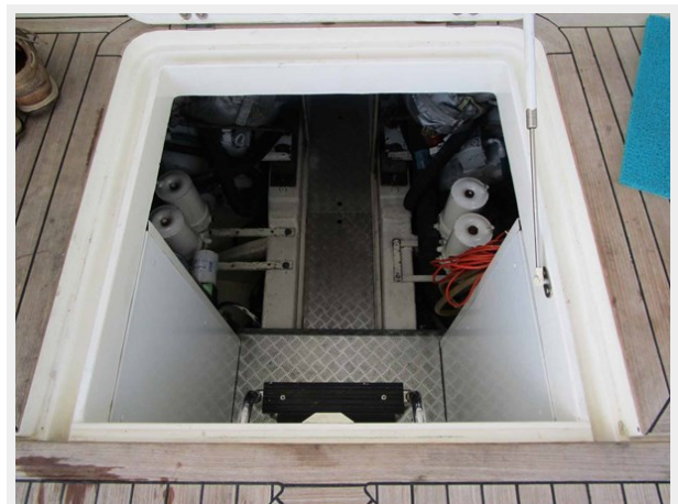
Engine Room Entrance
