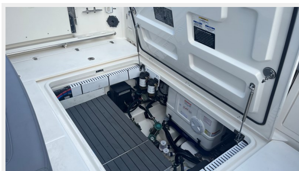
Generator and Aft Compartment
