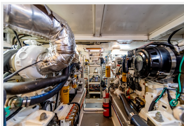
052 Engine Room SIERRA FOX 58_ Offshore
