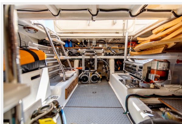
054 Engine Room SIERRA FOX 58_ Offshore
