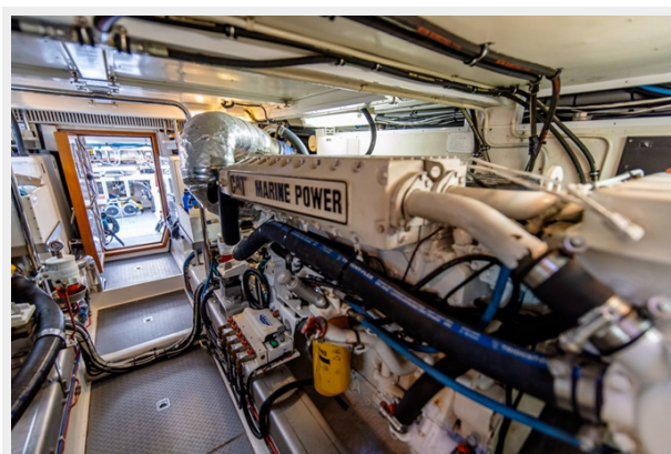
051 Engine Room SIERRA FOX 58_ Offshore
