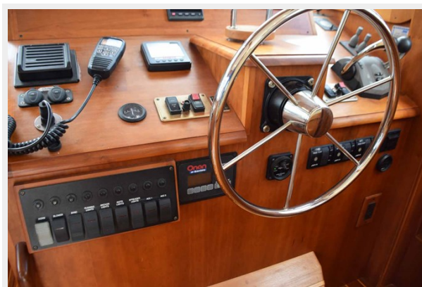
Lower helm switch panels
