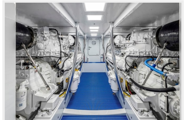
Engine Room-Forward View
