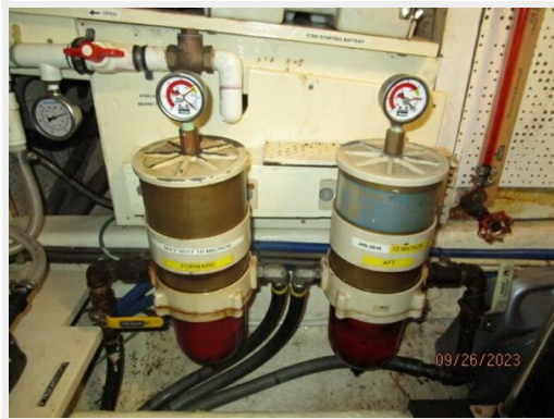
73_2803754_49_defever_racor_fuel_filters
