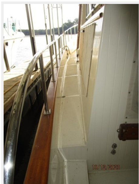
Pipe Dream port side deck2 10-12-23
