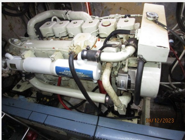
Pipe Dream main engine2 10-12-23
