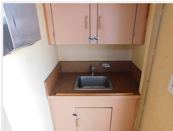
Commercial Fireboat - Galley
