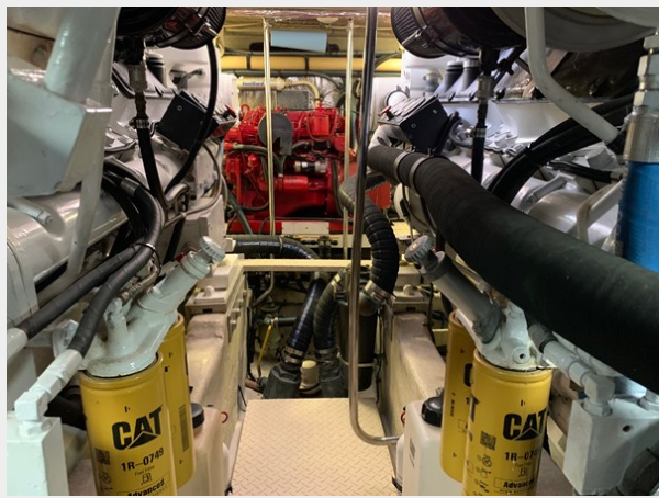
Engine Room CAT 3412's
