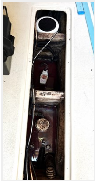
Fluxgate compass in bilge IMG_1780
