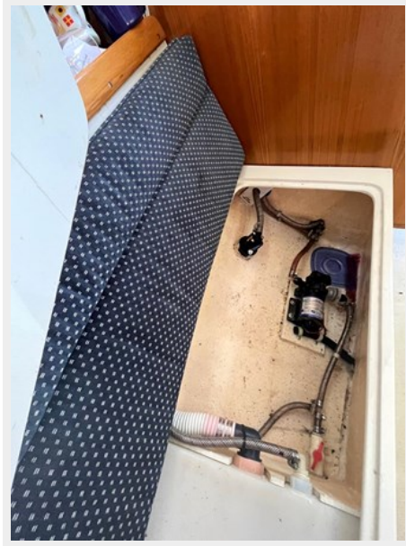
Freshwater pump IMG_1758
