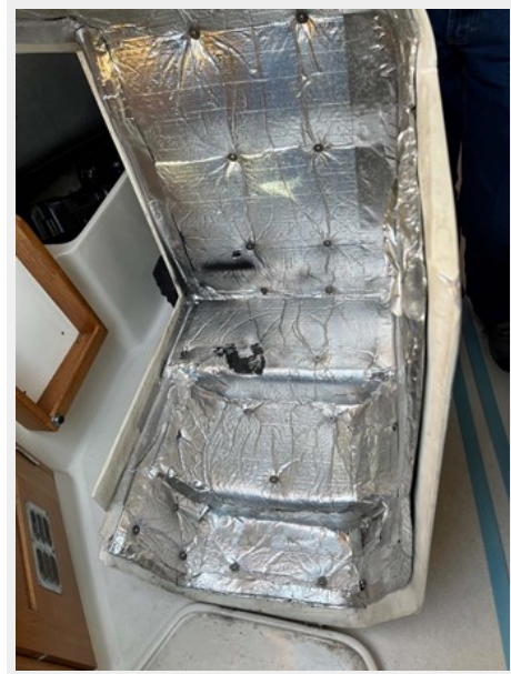
Engine insulation IMG_1782
