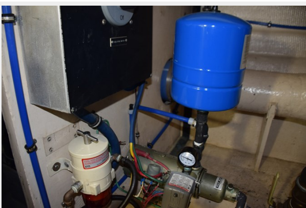
Rebuilt Freshwater Pump, New Accumulator Tank
