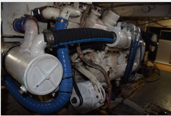
New Cooling Hoses and Many Fuel Lines
