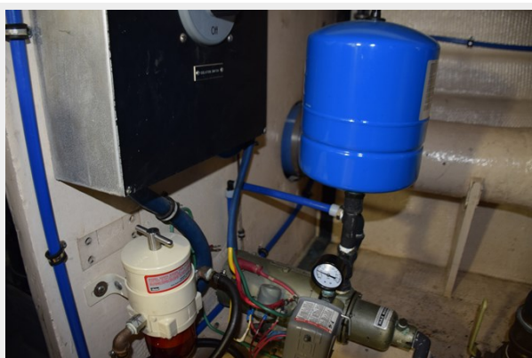
Rebuilt Freshwater Pump, New Accumulator Tank
