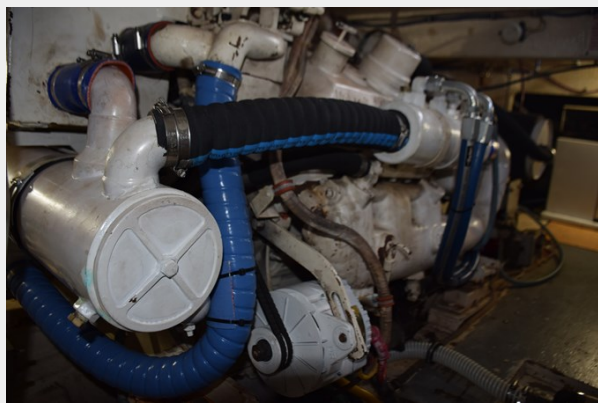
New Cooling Hoses and Many Fuel Lines
