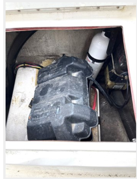
Battery & extinguisher - port aft IMG_2216
