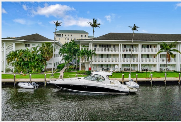
Final DJI_0381 -denoise-sharpen- enhance-8000w
