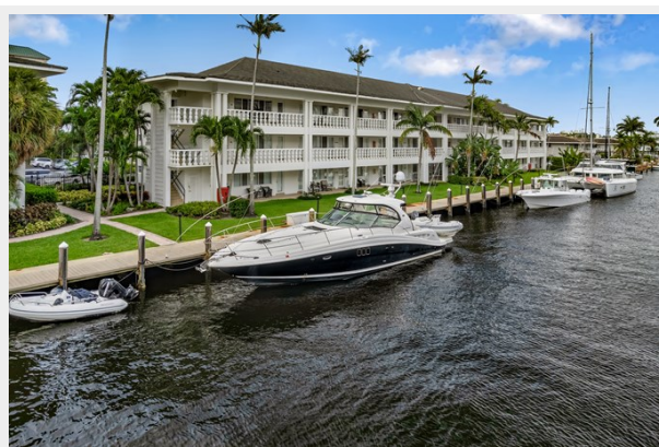
Final DJI_0377 -denoise-sharpen- enhance-8000w
