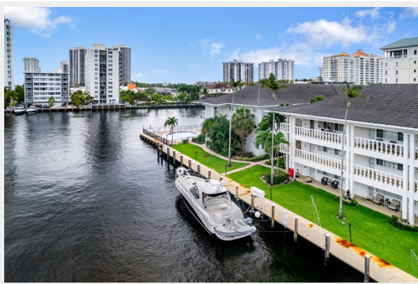
Final DJI_0410 -denoise-sharpen- enhance-8000w
