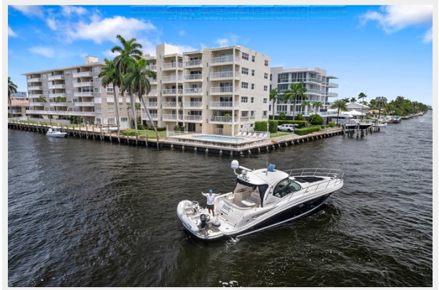
Final DJI_0468 -denoise-sharpen- enhance-8000w
