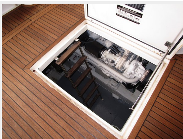
Engine Room Access
