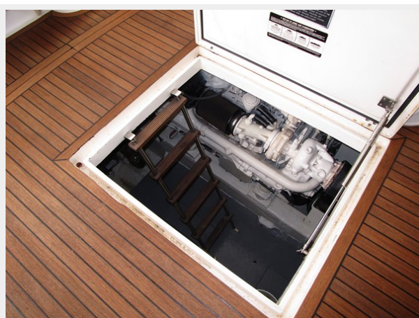
Engine Room Access
