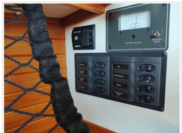
Phoenix Electrical panel
